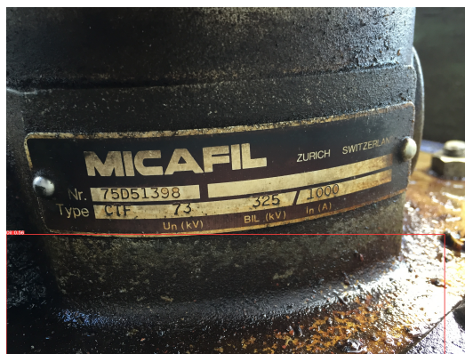
Figure 4.15: Oil Detection on Close-up Photograph
